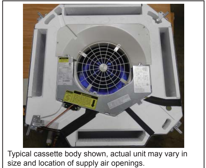
Figure 15. Typical Supply Air Configuration
