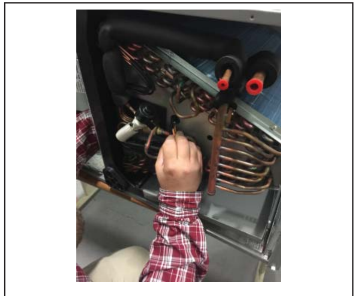
Figure 7. Coil Rotated 180°
