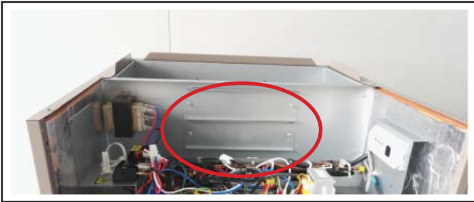
Figure 12. Remove Heat Kit Access Panel
