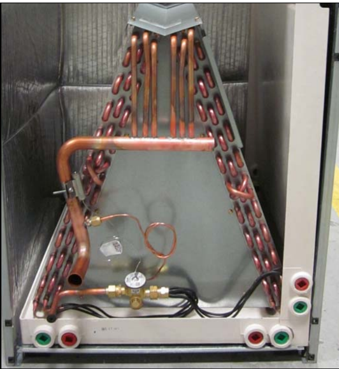
Figure 8. Slide Coil Assembly, Bottom Drain Pan and Horizontal Drain Pan Back Into the Air Handler as a Unit
