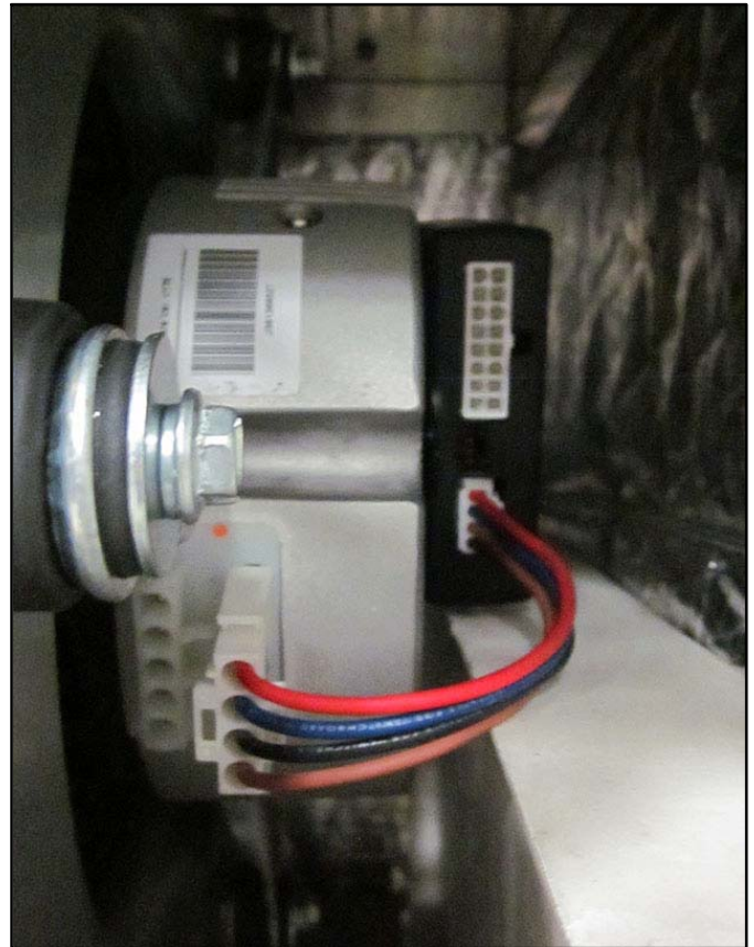
Figure 13. Blower Assembly Installed in Air Handler Cabinet with Required Clearance Between Horizontal Drain Pan and Motor Black Box
