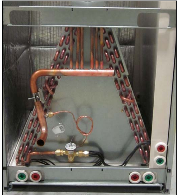
Figure 9. Reinstall Brackets that Hold the Coil and Horizontal Drain Pan in Place
