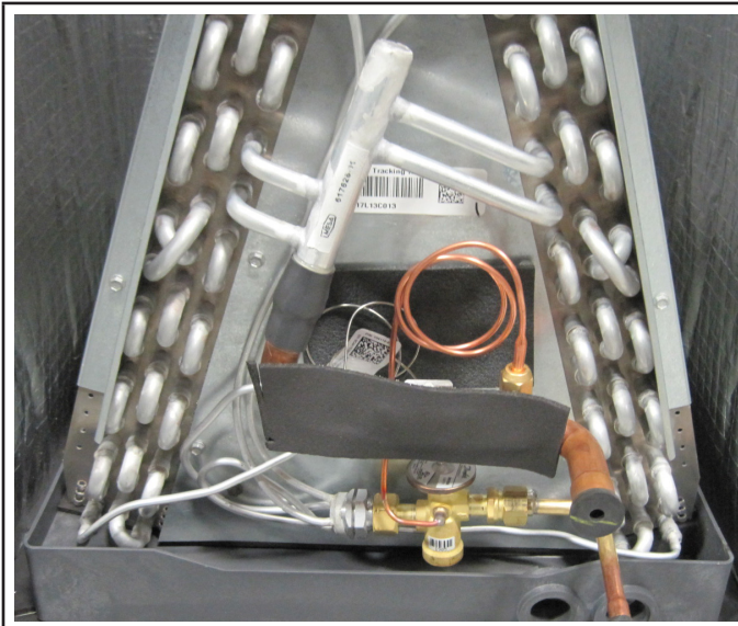
FIGURE 12. Insulated TXV Sensing Bulb
