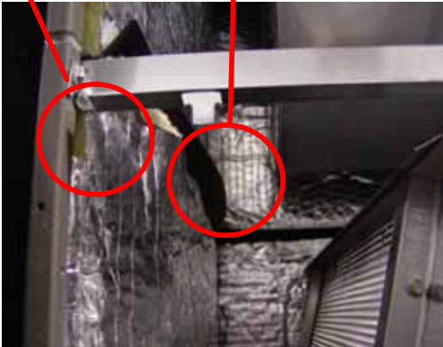
Figure 2. Cut Insulation and Improved Gasket
