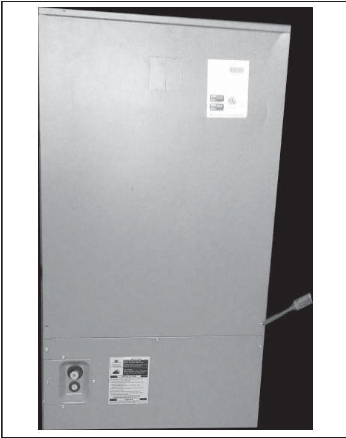
Figure 1. Remove Blower Access Panel
