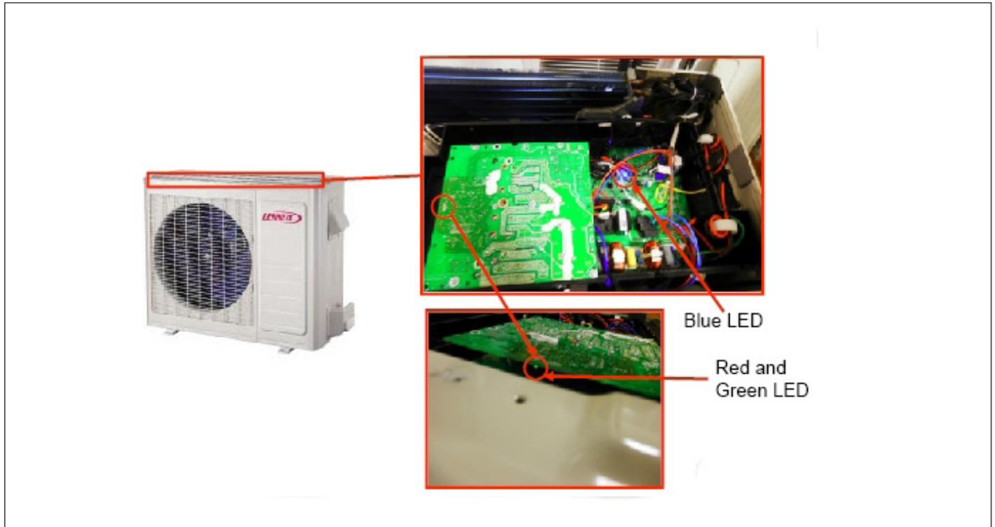
Figure 35. Typical Location of Outdoor Unit LEDs
