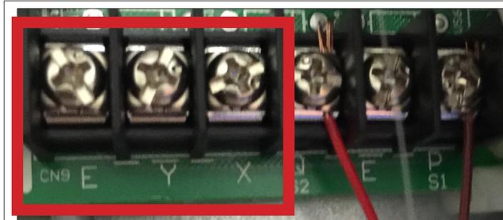
Figure 24. Typical Central Controller Connection Point Example 2
