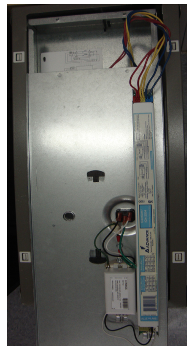
REMOVING ADVANCE BRAND BALLAST AND LENNOX SURGE PROTECTOR
