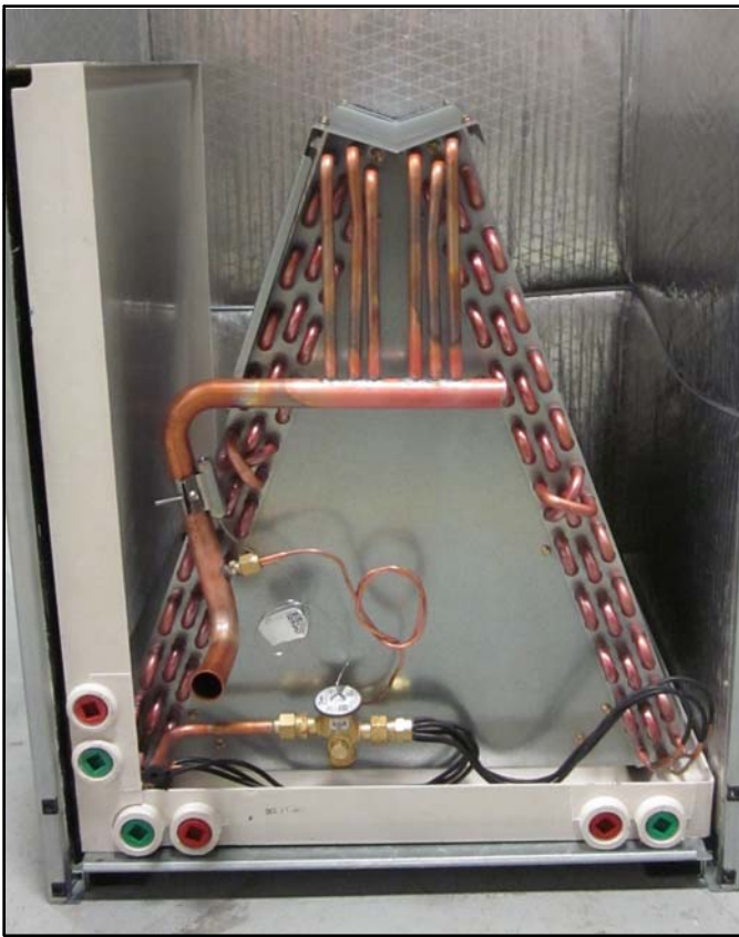
Figure 19. Remove Coil Assembly, Bottom Drain Pan and Horizontal Drain Pan as a Unit
