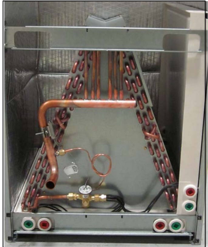
Figure 30. Reinstall Brackets that Hold the Coil and Horizontal Drain Pan in Place
