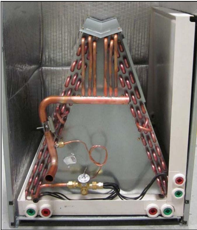
Figure 29. Slide Coil Assembly, Bottom Drain Pan and Horizontal Drain Pan Back Into the Air Handler as a Unit
