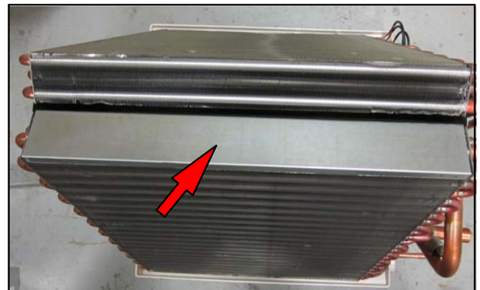
Figure 27. Remove Blow-Off Prevention Brackets, Top Cap and Drip Pan
