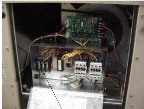
CONNECT LINE VOLTAGE (PIVOTING CONTROL BOX SHOWN)
